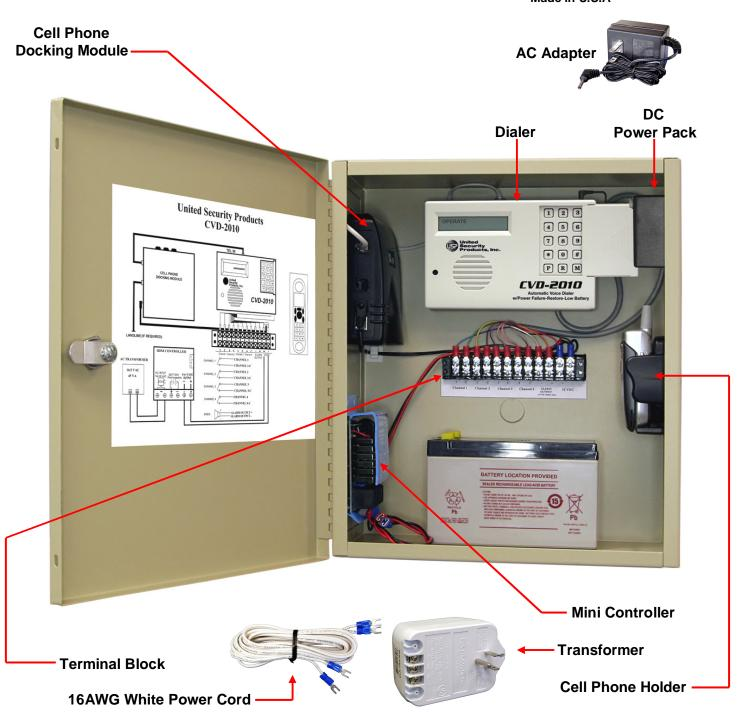
Cell Phone included with CVD-2010P and CVD-2010PS Battery not included with Systems
